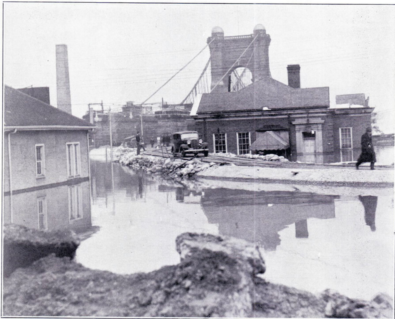
Covington end of Suspension Bridge.
