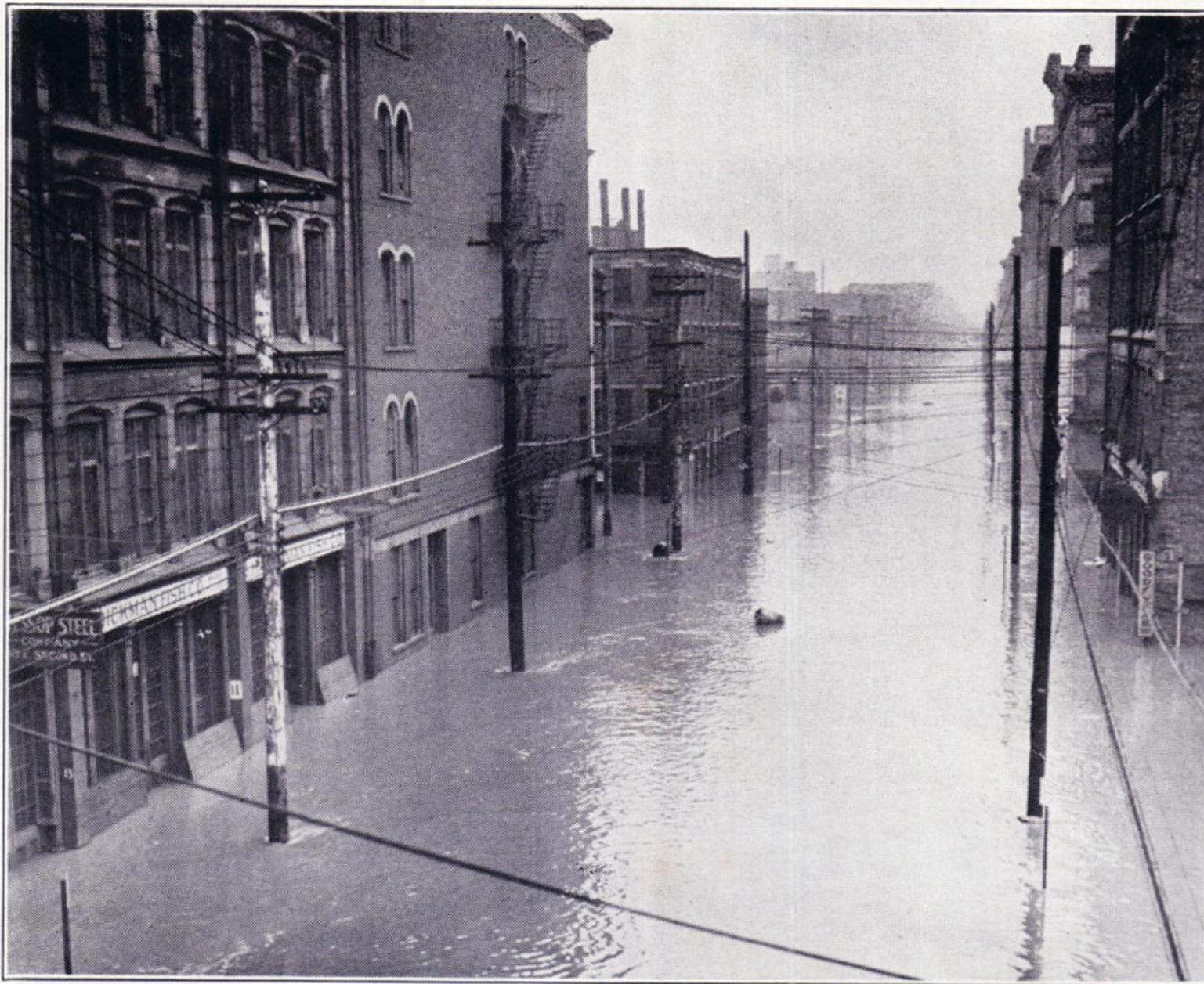
Scene on East Front Street, in Cincinnati's wholesale merchandising district, when the Ohio approached the flood crest.
