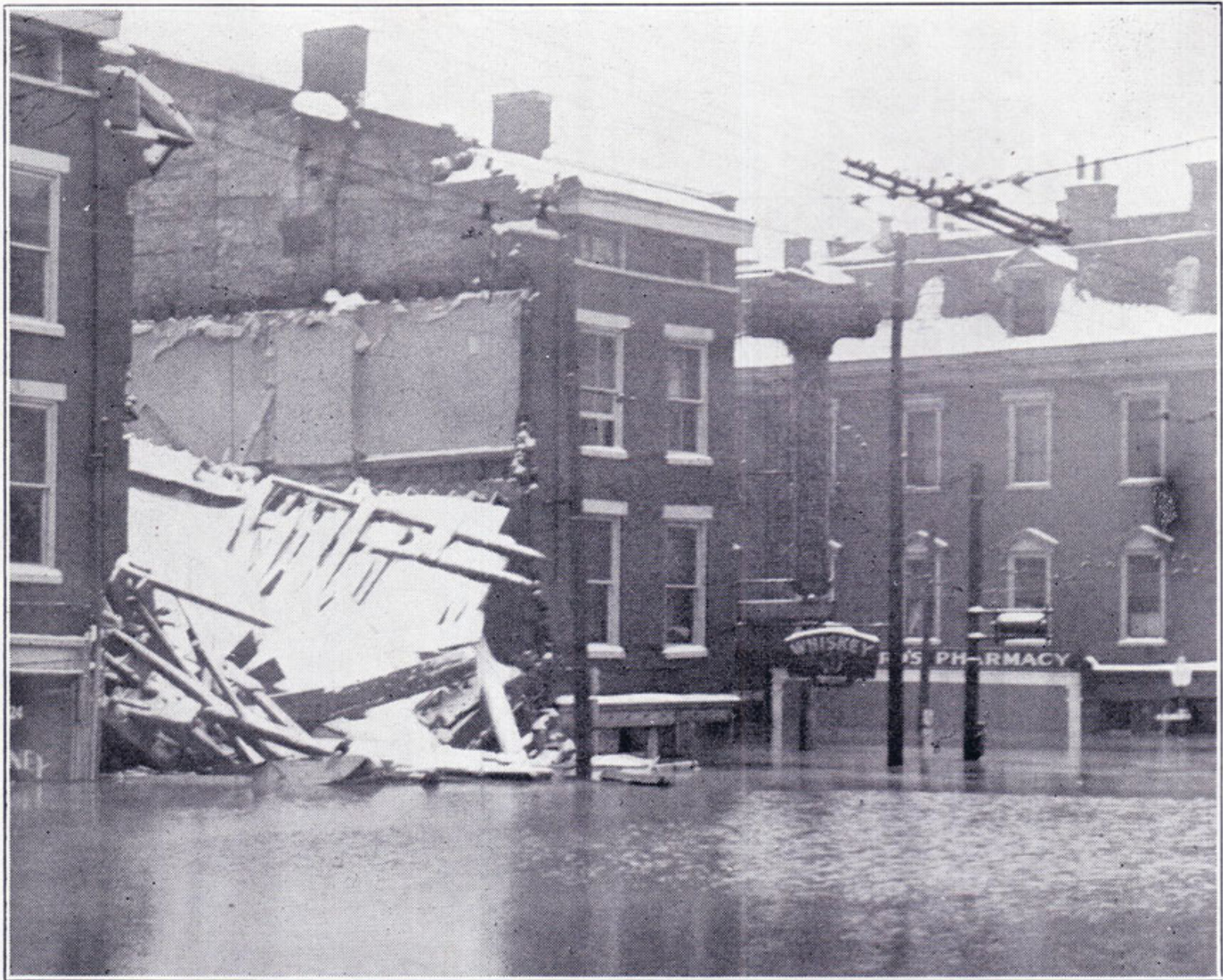
Building which collapsed in flood waters of the downtown section, Third and Broadway. Six families escaped to the roofs and were lowered by ropes to the street.
