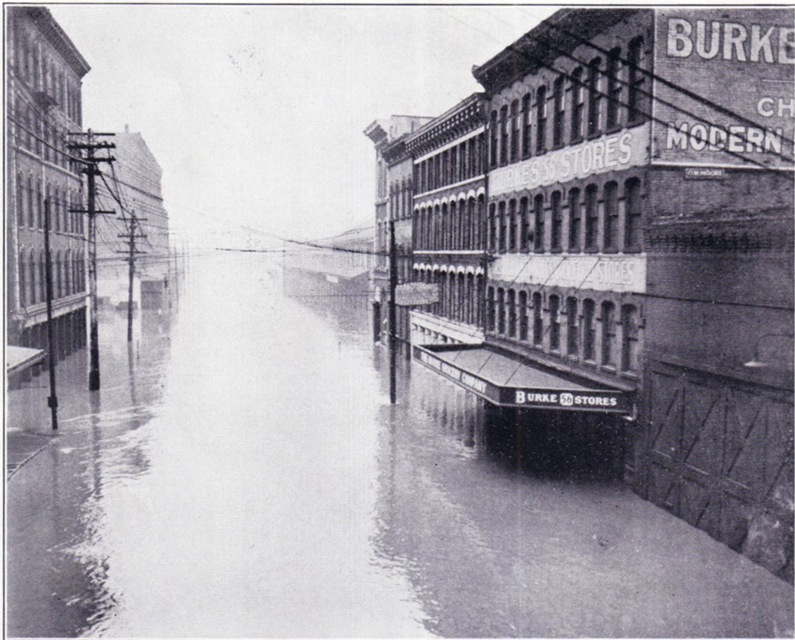
Looking west on Second Street from Suspension Bridge.
