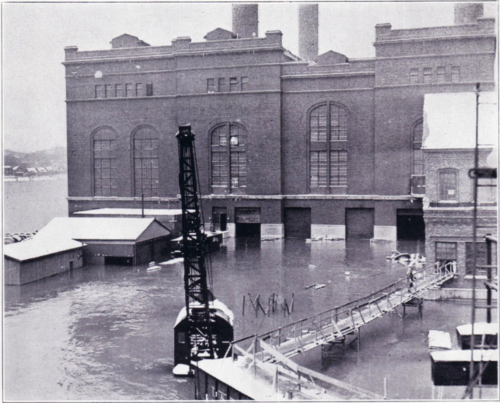
Cincinnati Gas and Electric Plant, Front and Rose Streets.
