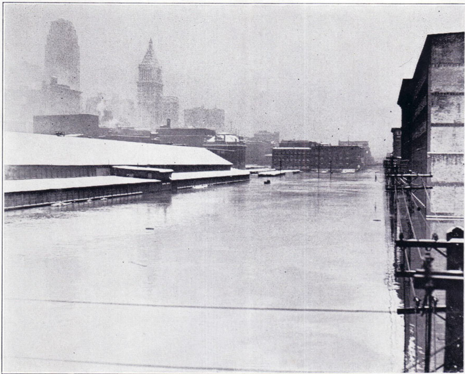
Looking east on Second Street from Smith Street, at the Bridge.
